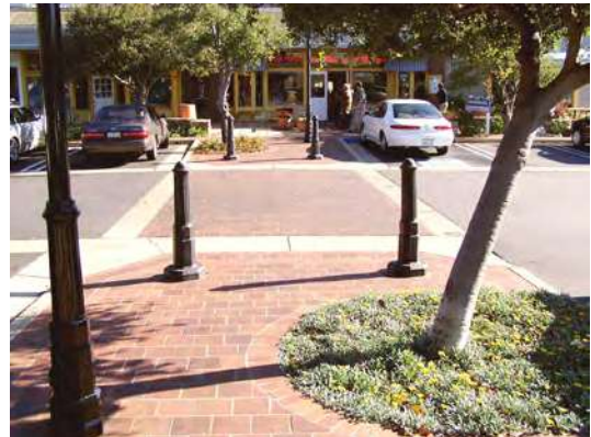
Raised intersection – location unknown
