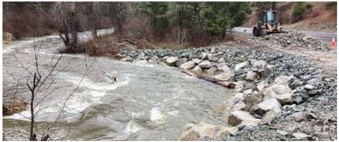
Bank stabilization on SR 21
