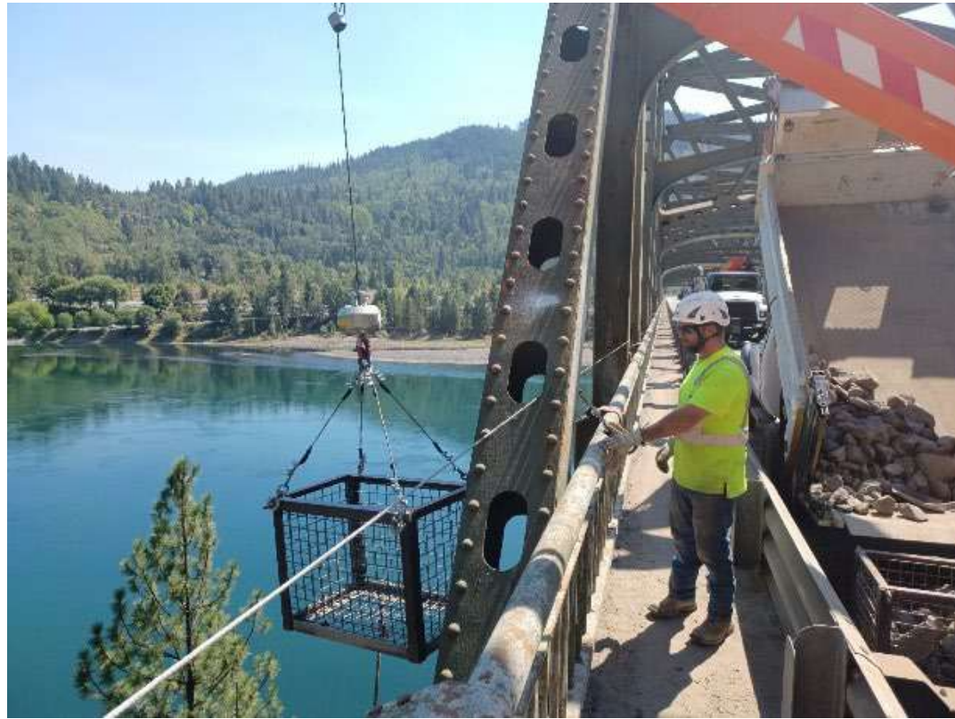
Erosion control on SR 25/Northport
