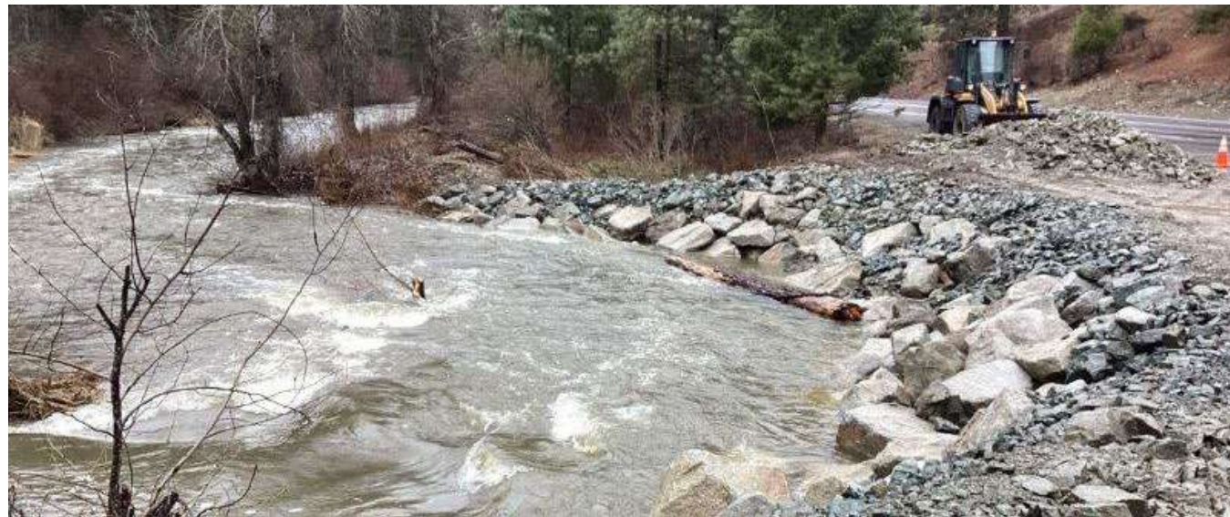
Bank stabilization on SR 21
