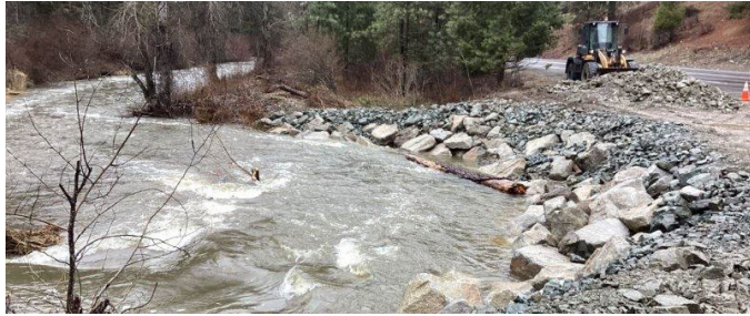
Bank stabilization on SR 21
