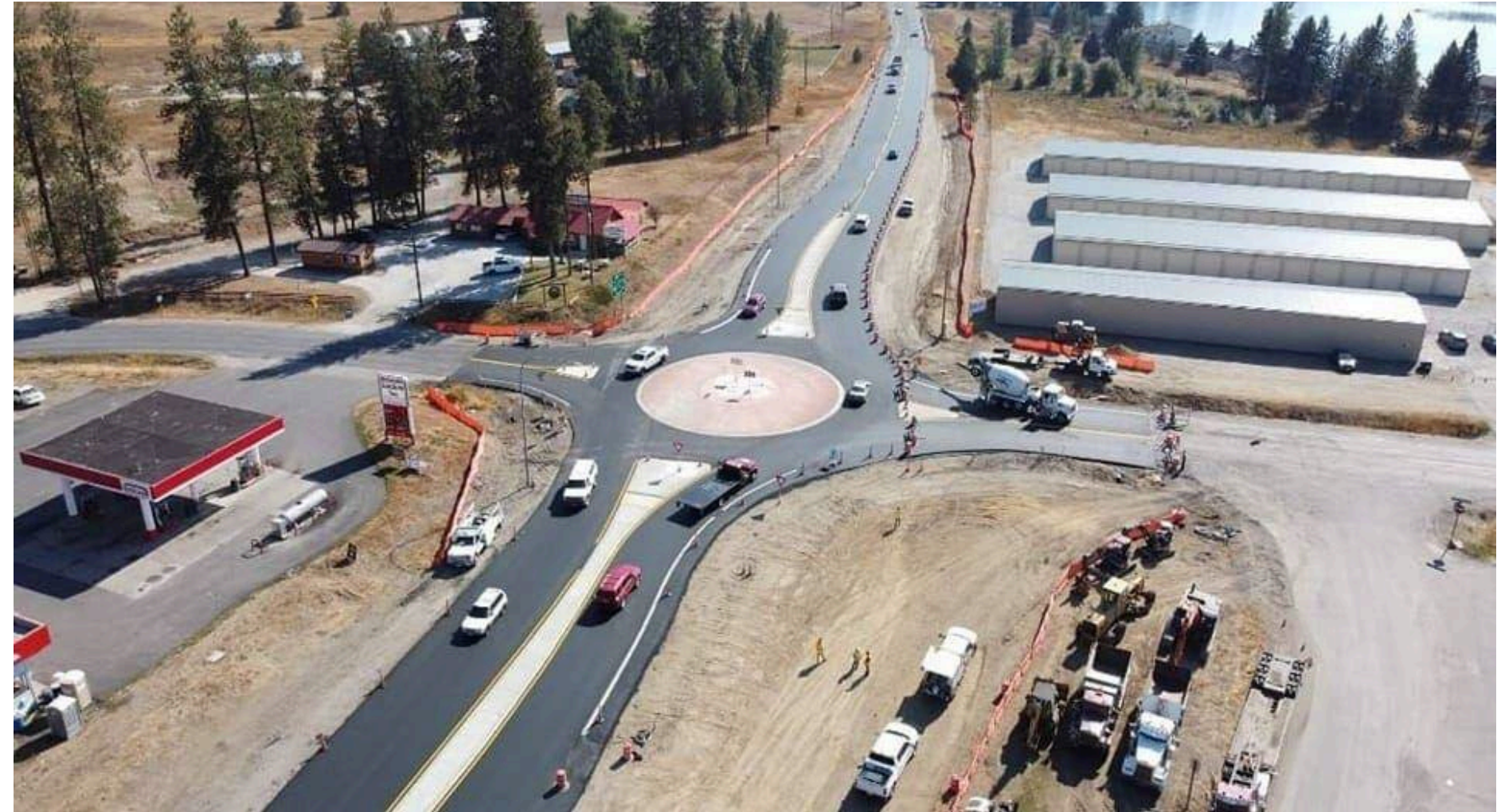
Compact roundabout added at US 395 and State Route 292 interchange in Loon Lake due to previous collisions.
