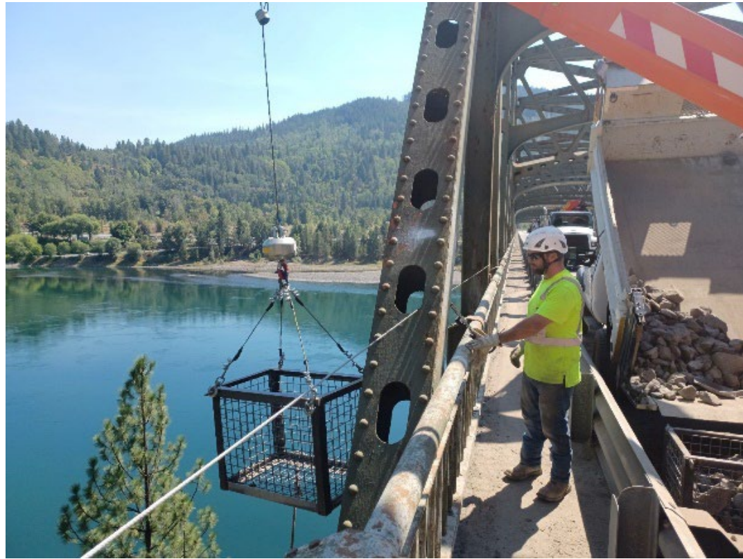
Erosion control on SR 25/Northport
