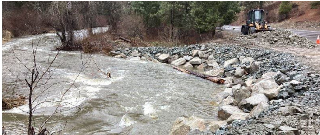
Bank stabilization on SR 21
