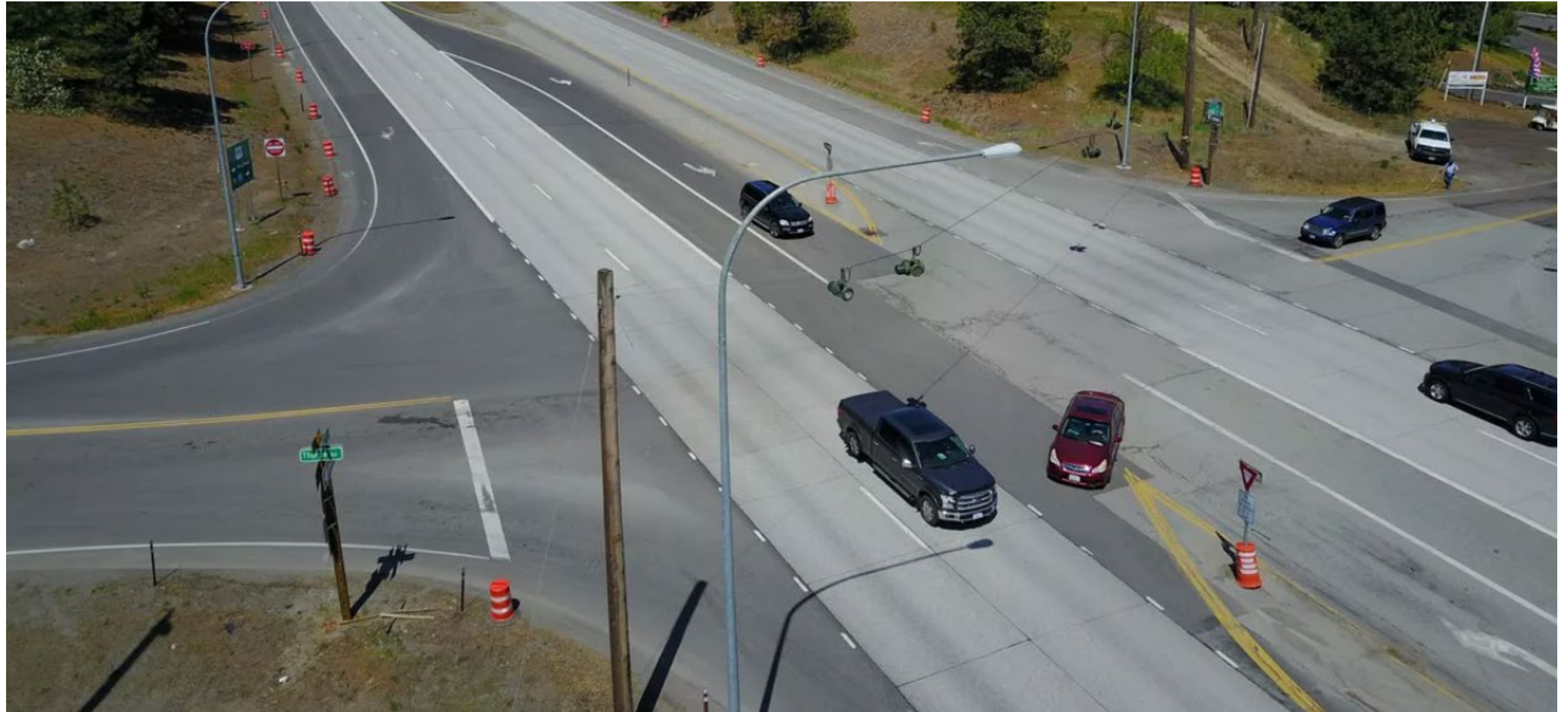
US 195 & Thorpe Road prior to J-Turns in 2019
